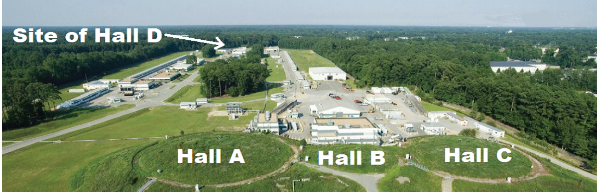
Figure 1: A view of JLAB showing the locations of experiment halls A through D. ( http://blogs.umass.edu/miskimen/files/2012/08/jlab.png )
