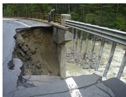
Fig. 7. Examples of common erosional impacts to the Deerfield River watershed from Hurricane Irene.
